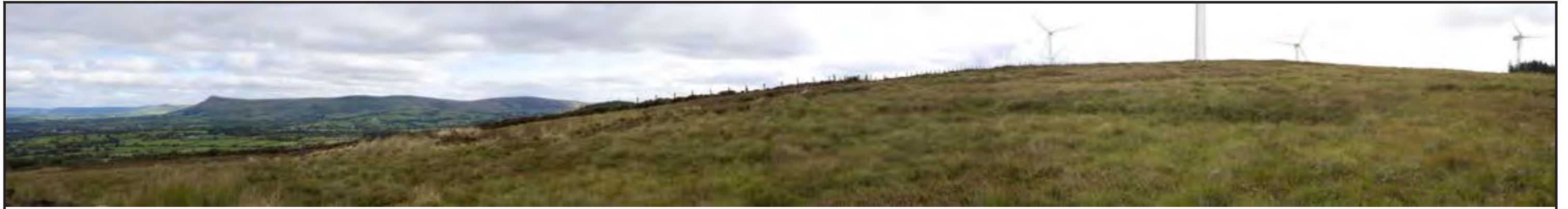
Extent of view from south east to north east of Magheramore Wind Farm
